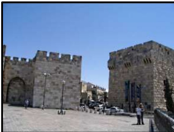
Jaffa Gate a century ago and today with road access
